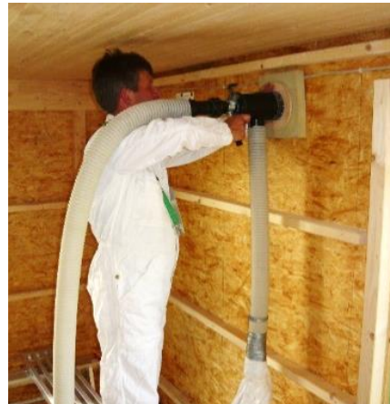
Figure 5: Cellulose insulation in walls
