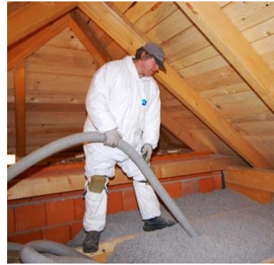
Figure 3: Cellulose insulation in open attics
